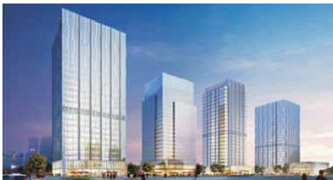
东莞寰宇汇金大厦 Dongguan Huanyuhuijin building 62层/站 7.0m/s
