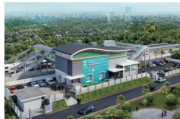
Indonesia Metland Telaga Murni Station Project
